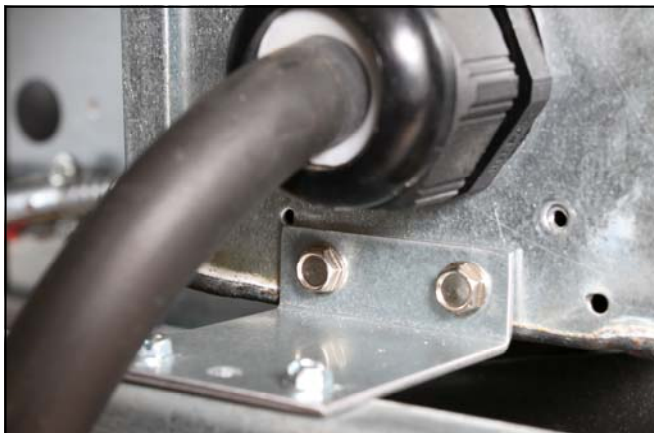
Figure 9: (Center-Mounted Contactor Box) Position the provided contactor box bracket, as shown. Use cabinet screws to attach it to the contactor box and provided drill-point screws to secure it to the cabinet channel.
