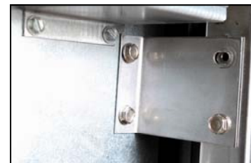
Figures 2 (left) and 3 (above): The existing contactor box brackets are shown left and above. They are replaced if they are below a linear actuator to be replaced.
