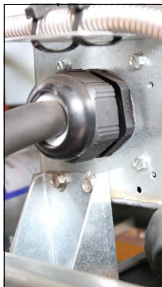
Figures 2 (left) and 3 (above): The existing contactor box brackets are shown left and above. They are replaced if they are below a linear actuator to be replaced.
